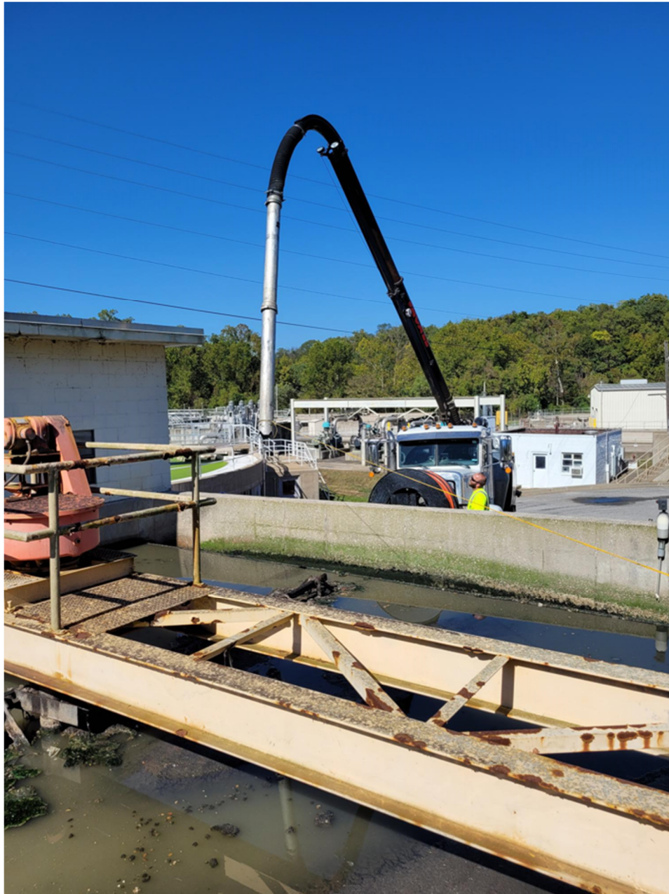
Existing Grit Basin cleaning on October 15, 2025
